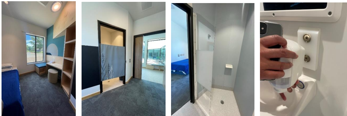
Mokopuna bedrooms and example of anti-ligature fixtures and fittings
